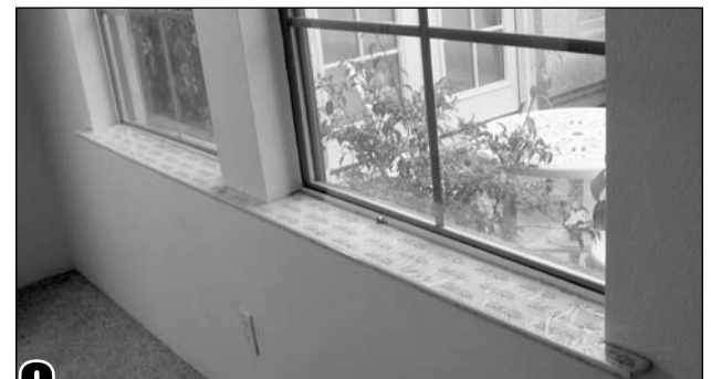
9 Remove the shims and set the Sill-Rite sill in the openings. Check for fit and adjust as necessary. Finish installing by following steps 8-11 of the Basic Installation Instructions .
