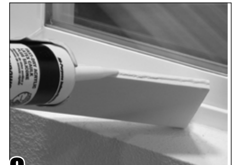
9 Apply a bead of caulk to the back edge of the sill.
