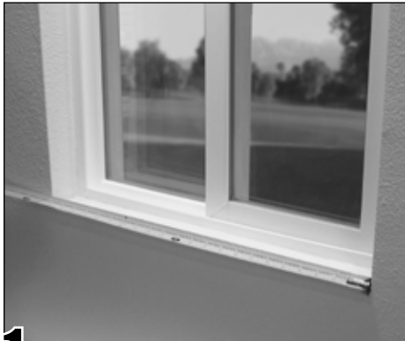
1 Measure the width of the window opening from jamb to jamb.
