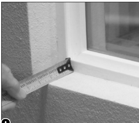
2 Measure the depth of the window opening in three places (each end and the center). Note the largest of these dimensions.
