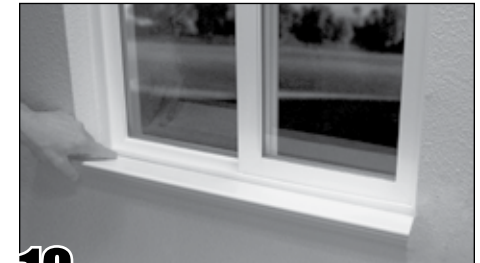
10 Insert the sill at a slight angle making contact with the window, then pivot the sill down in place.
