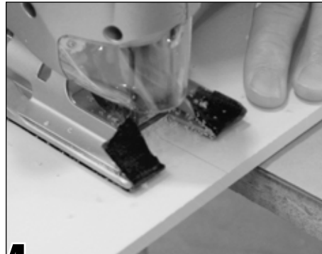
4 Cut the sill to the width of the opening.
